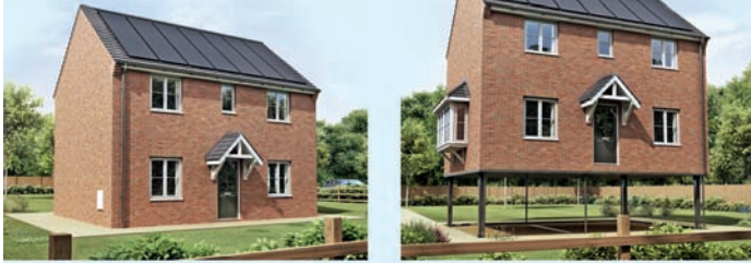
The Larkfleet 'elevating house' – at normal height and elevated on jacks in advance of flooding.
